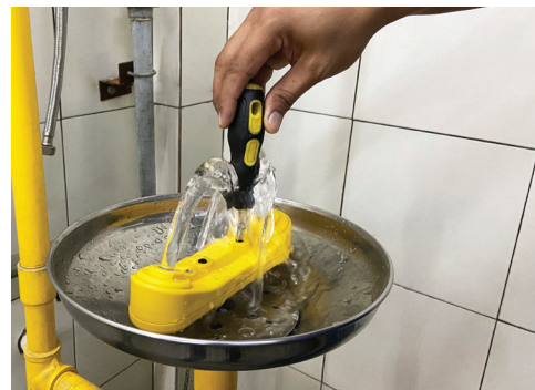
Manually regulate flow to ensure steady stream regardless of pressure
